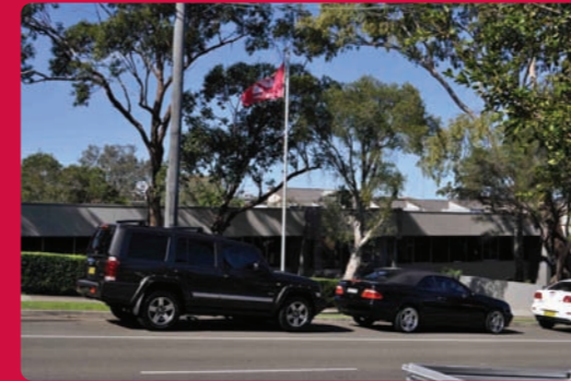
East Facing view of Assetlink support office
